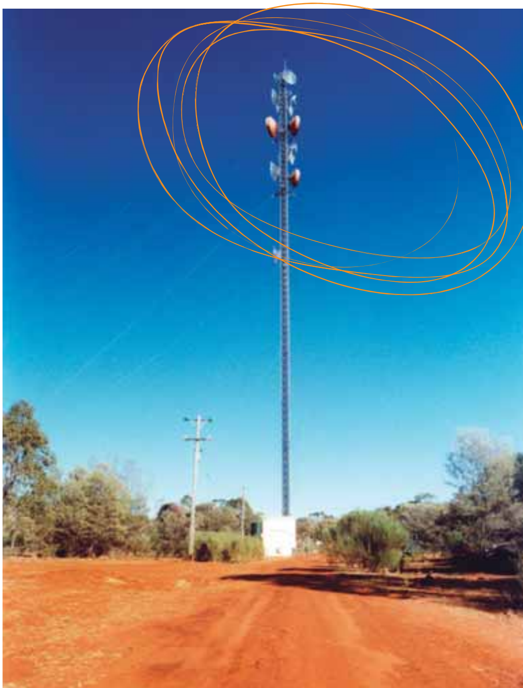
Rosewood radio tower north of Augathella in western Queensland.
