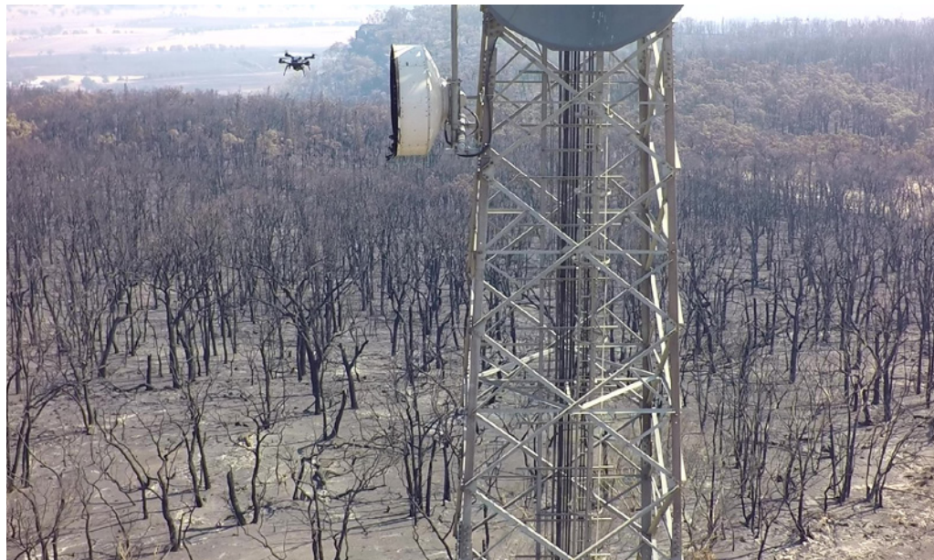
Taken near Broombee NSW, during times of crisis, drones can provide faster inspections of our infrastructure so that we can keep communities connected when they need it most.
